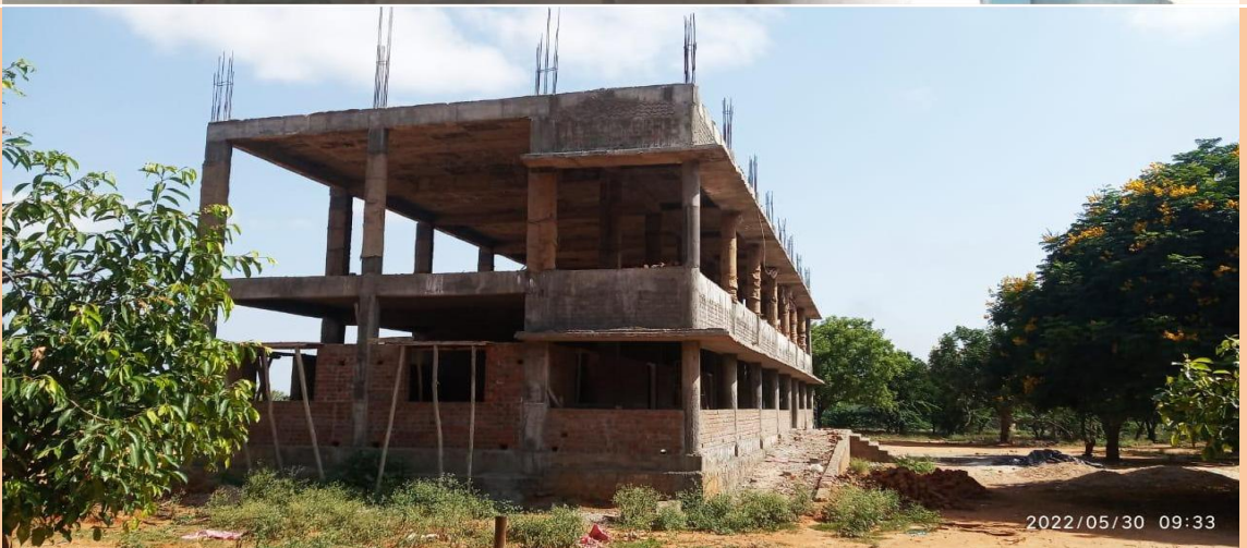
Construction of New Classrooms Block
