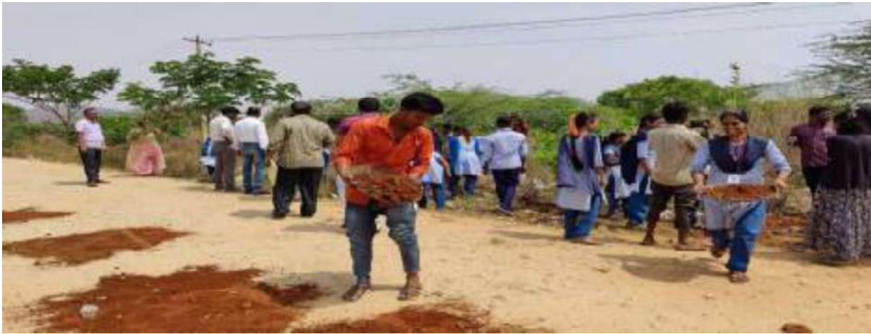
Filled with Gravel and sand on the road pits
