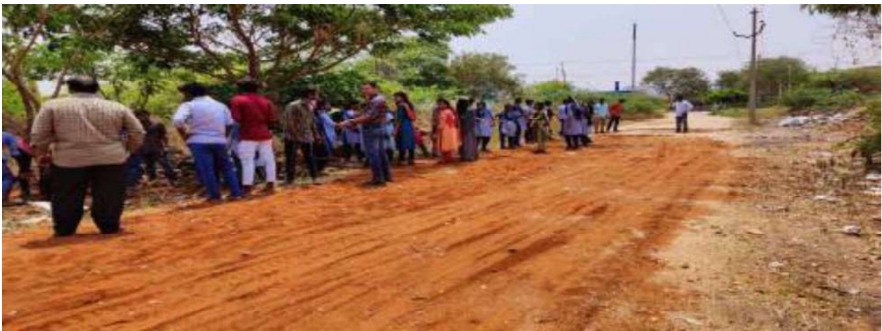
Students and Staff at repairing the ROAD
