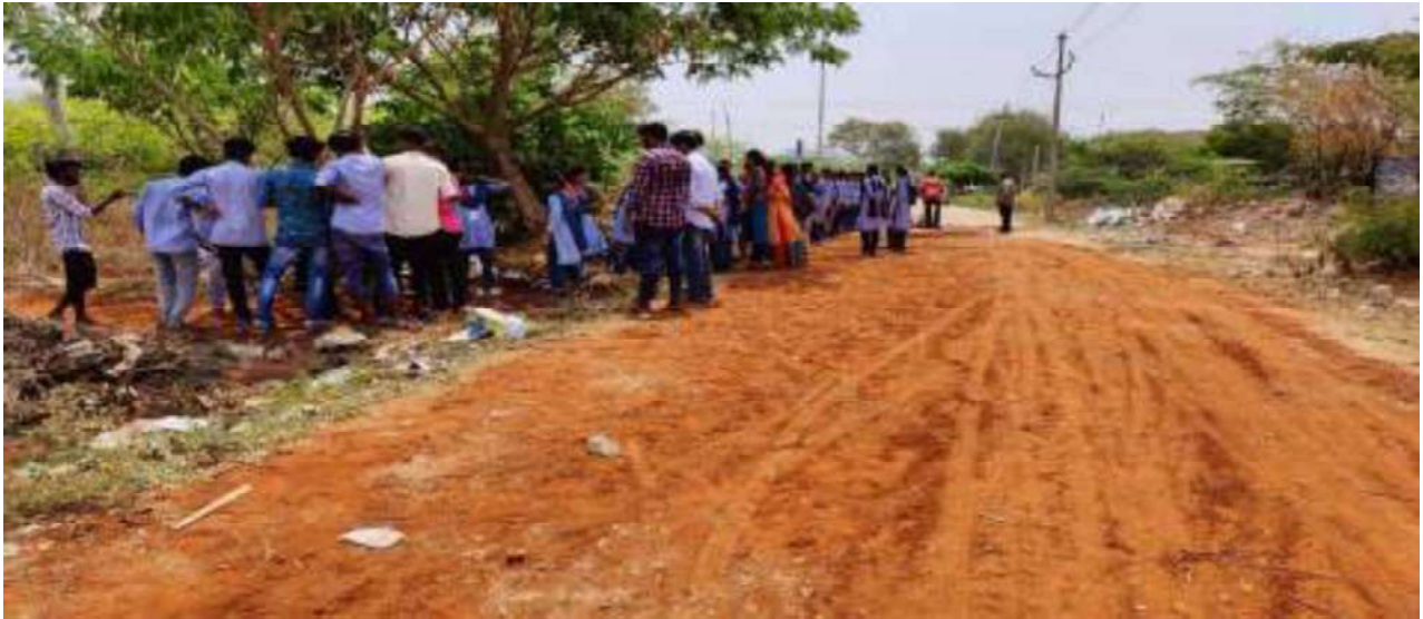
After Repair the Road
